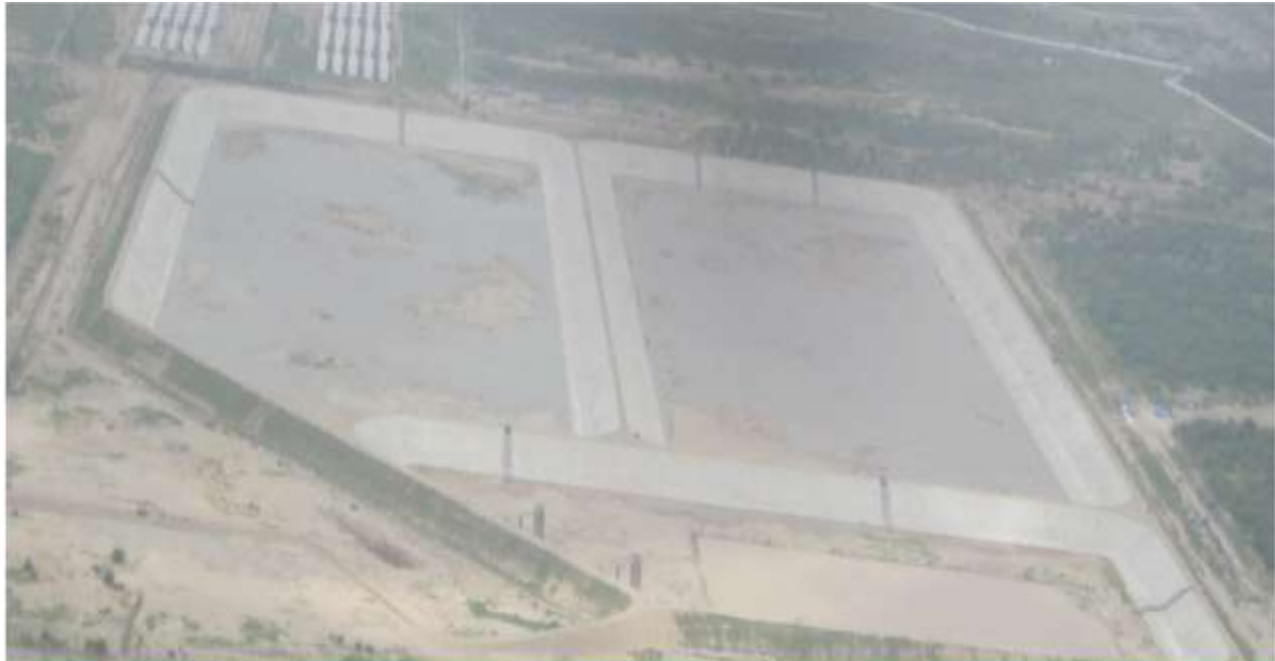
HDPE impervious Lined Ash Pond to avoid ash water ingress into ground
